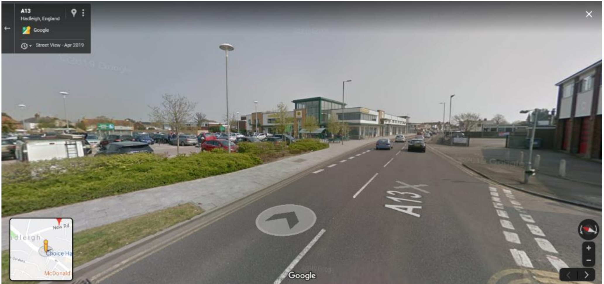
Photo facing south east bound on the A13 London Road, showing the proposed location of new exist slip which will direct traffic back on to the A13 London Road
