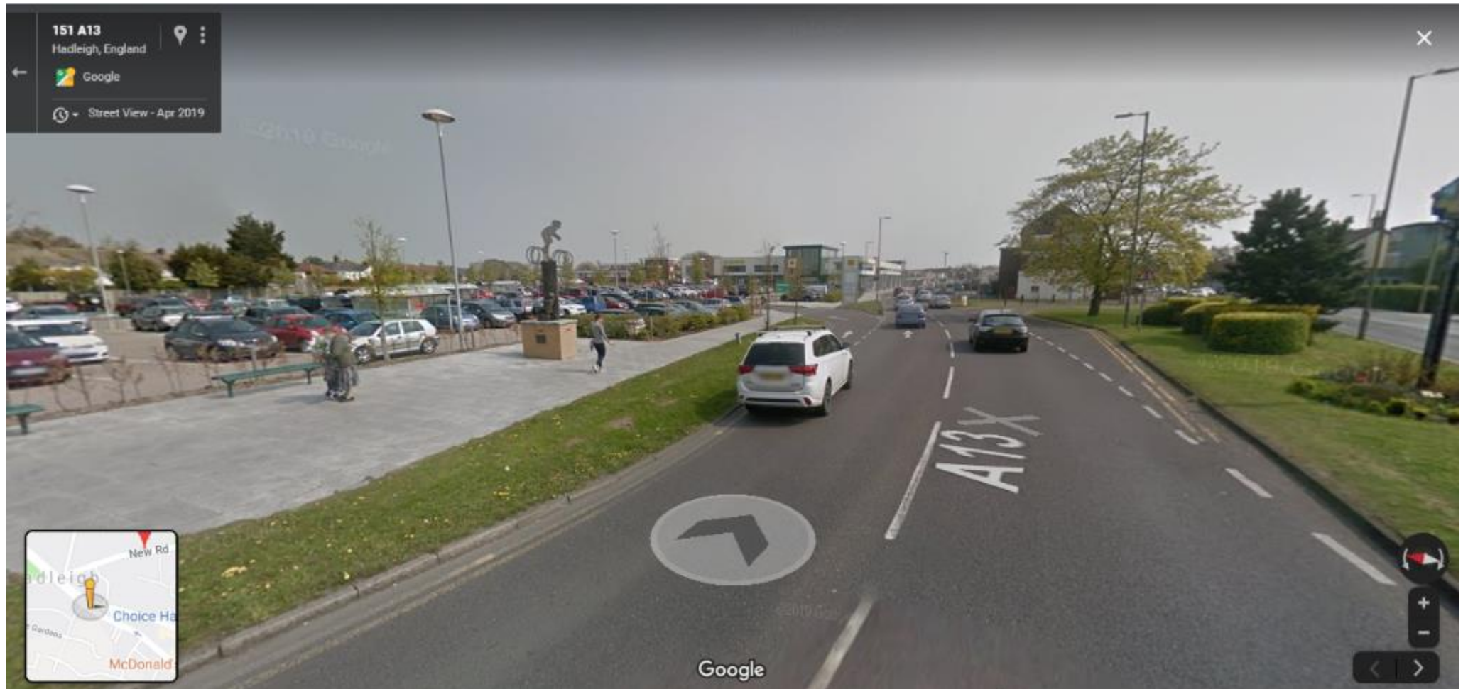
Photo facing south east bound on the A13 London Road, showing the start of existing entrance slip to Morrisons carpark
