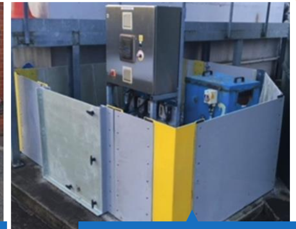
J-Bar flood barrier around critical equipment with swinging barrier at Gosfield Water Recycling Centre
