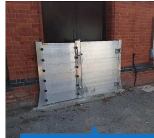
Flood swinging barrier and stop logs at Bocking Water Treatment Works.
