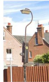
Fig 1 – Isolation box and lantern on cast iron column
