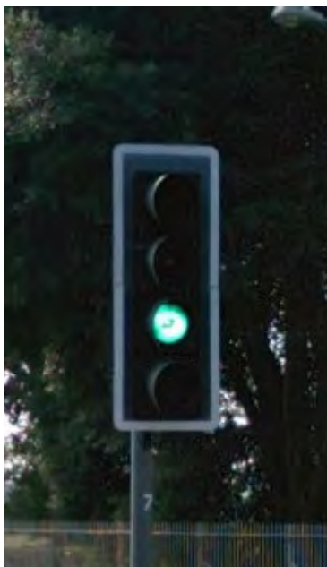
Existing secondary head on Mersea Road for right turning traffic with indicative green situated below the "normal" green aspect.
