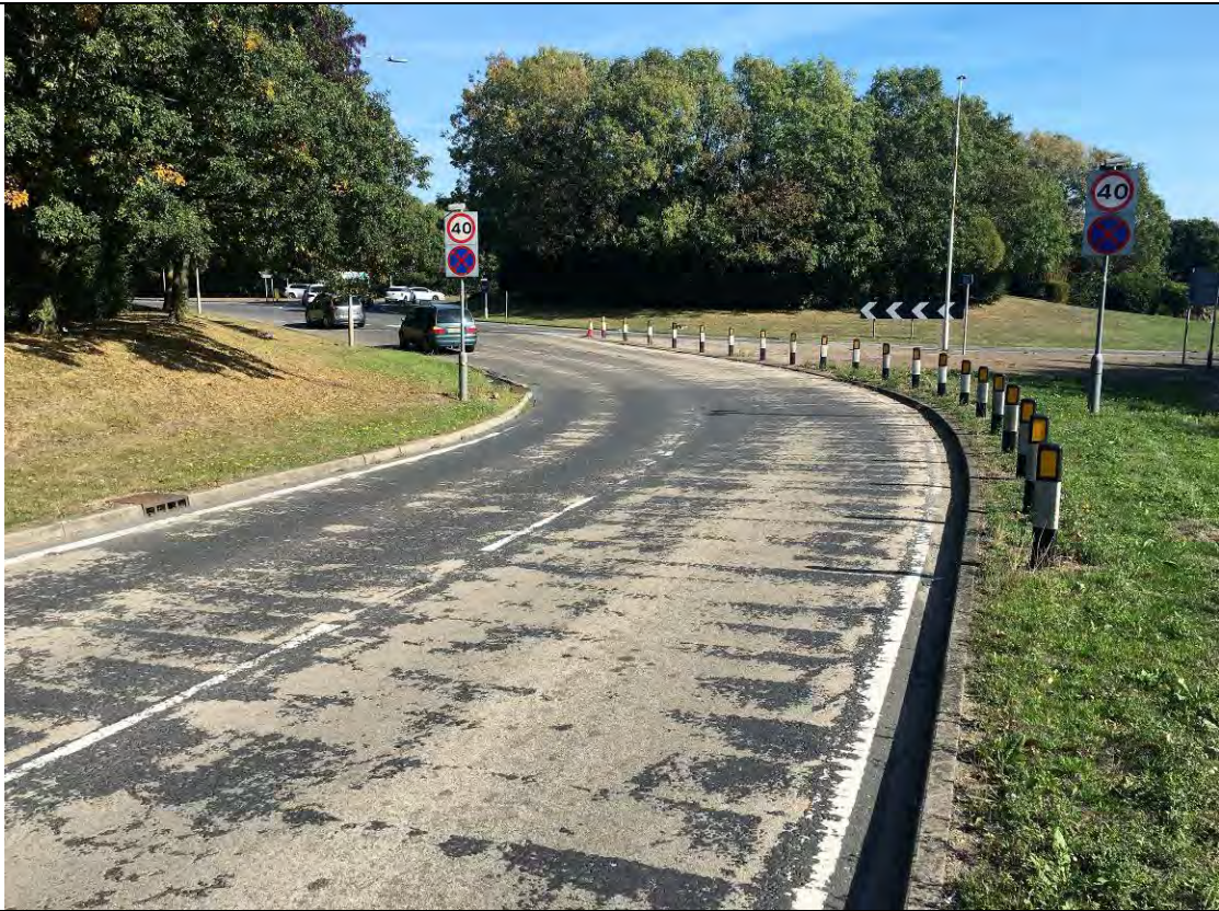
Image 2 – 40mph speed limit signs & clearway signs on the eastbound approach. Worn edge of carriageway and centre line road markings.
