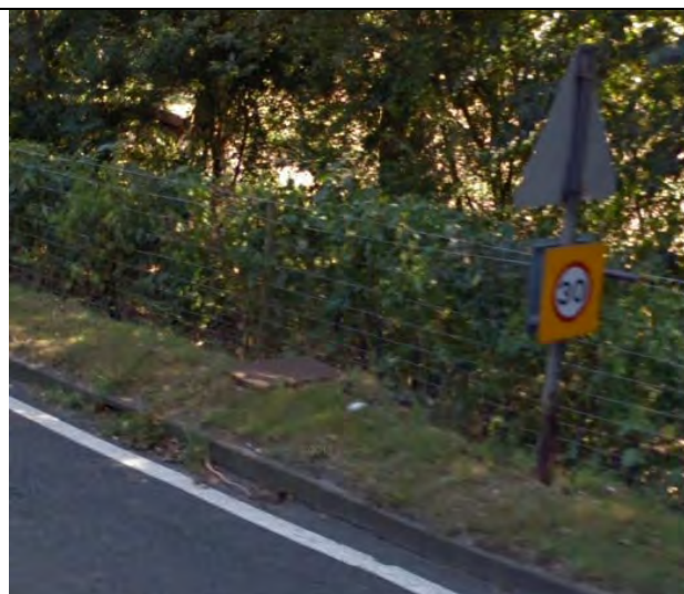
Existing gulley offlet south east of the bend likely to be piped into adjacent field.
