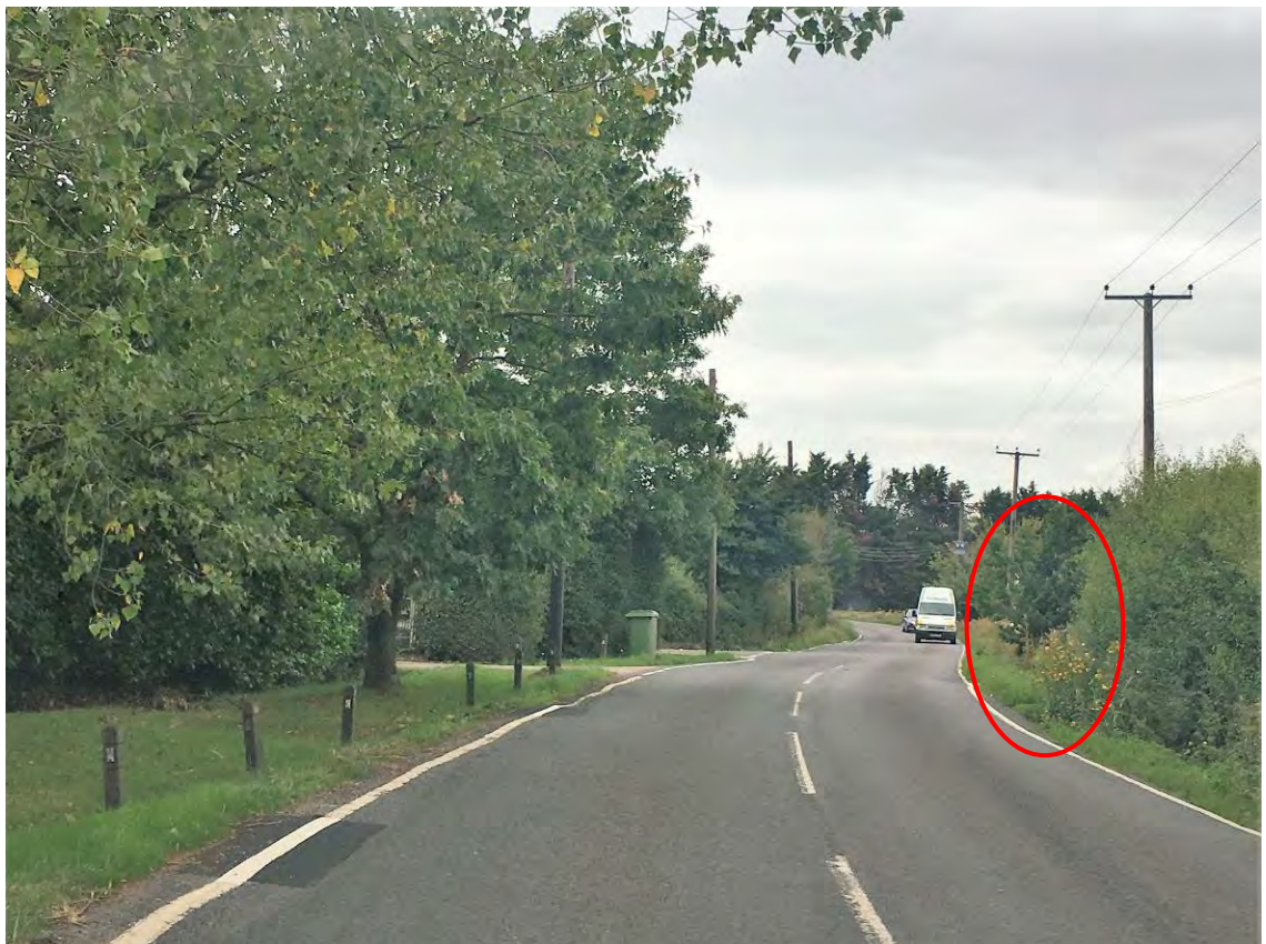
Image 7 – Overgrown vegetation to the northern side of Thoby Lane restricts forward visibility to the existing finger post directional sign opposite St Annes Road
