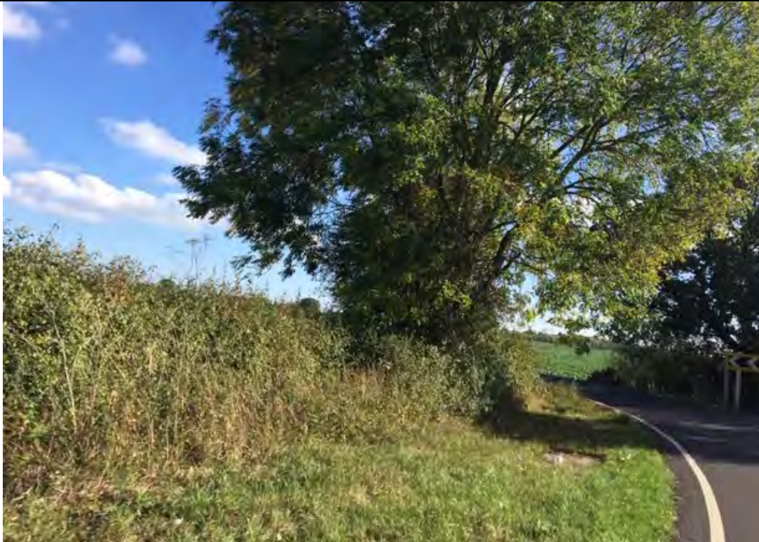
Image 2 – Vegetation within inside of southernmost bend obstructing forward visibility
