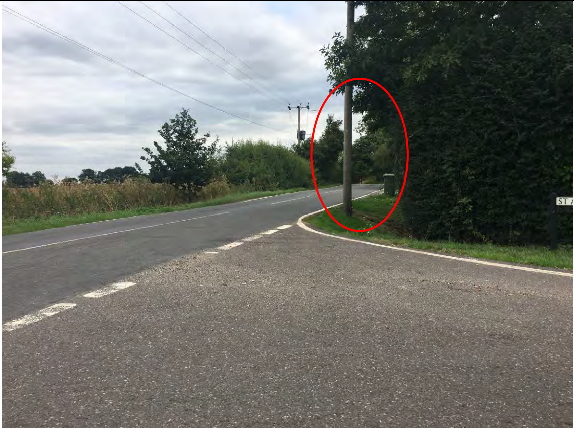
Image 6 – Telegraph pole and overgrown vegetation located the within visibility splay to the right when sitting in at the give way lines on St Annes Road
