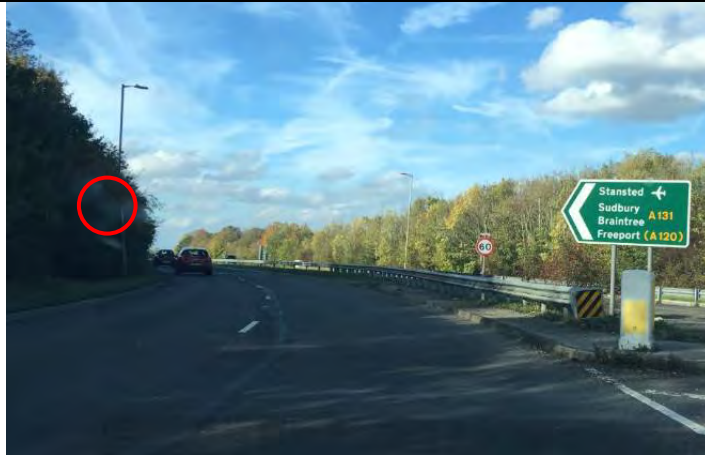
Image 3 – View looking north leaving the roundabout circulatory. Image shows missing nearside 60mph Terminal
