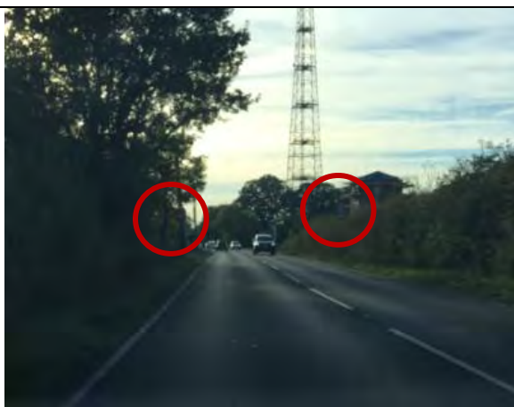
Image 11 – View looking South/West on Halstead Road with the change in speed limit (circled in red), note the speed limit signs do not stand out against the back ground.
