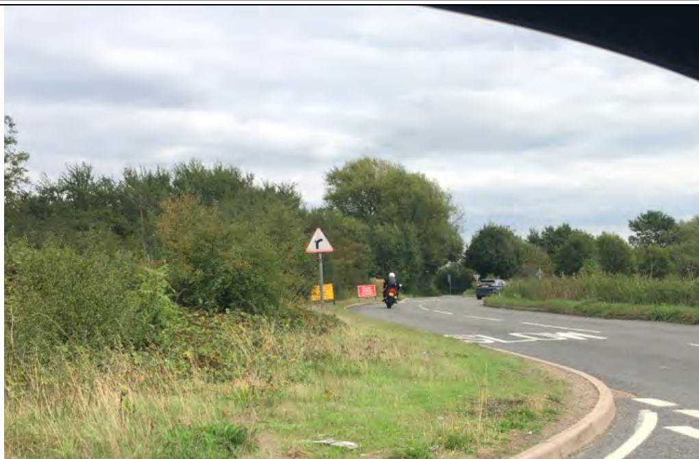
Image 1 – Existing ‘Side road on bend ahead’ warning sign on Wash Road / Widvale Road eastbound approach is partially faded
