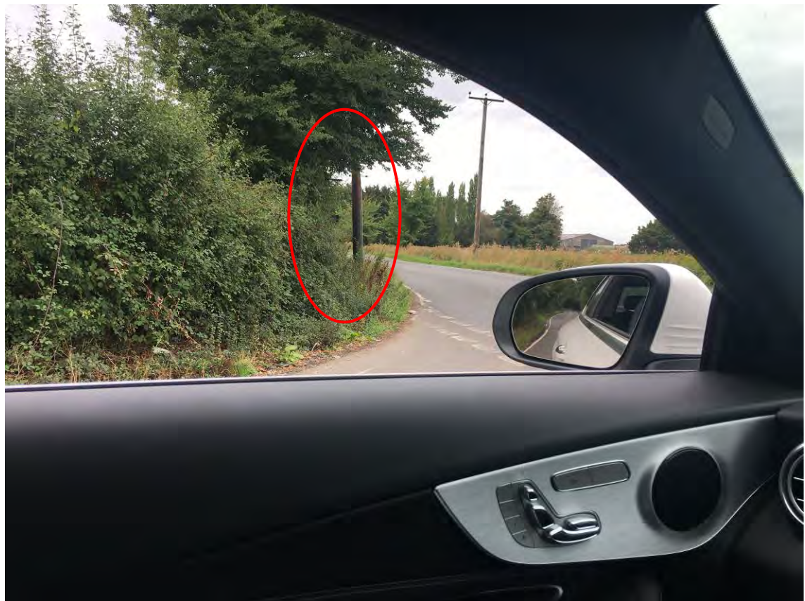
Image 5 – Telegraph pole and overgrown vegetation located the within visibility splay to the left when sitting in at the give way lines on St Annes Road
