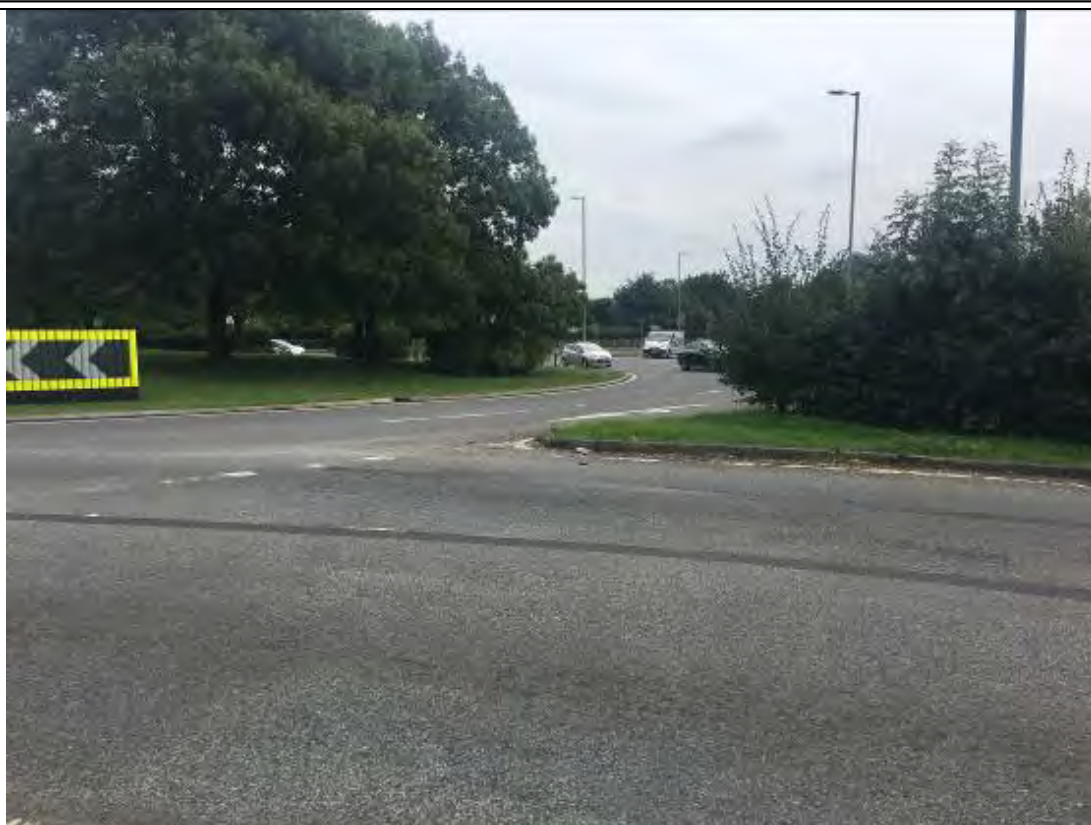
Image 1 – Existing highway screening / hedgerow terminates immediately adjacent the give way lines, impeding the visibility splay for eastbound motorists
