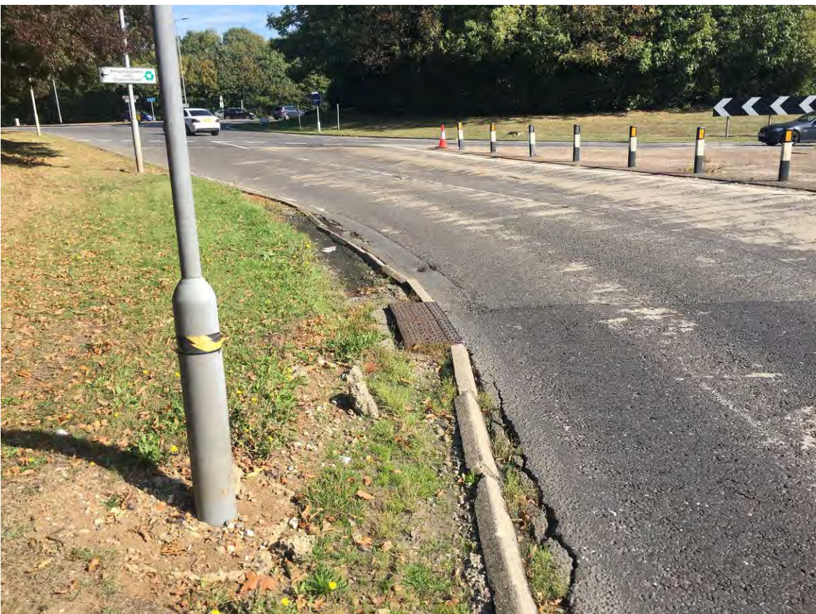
Image 6 – Lane line road marking obscured by joint repairs on northbound approach
