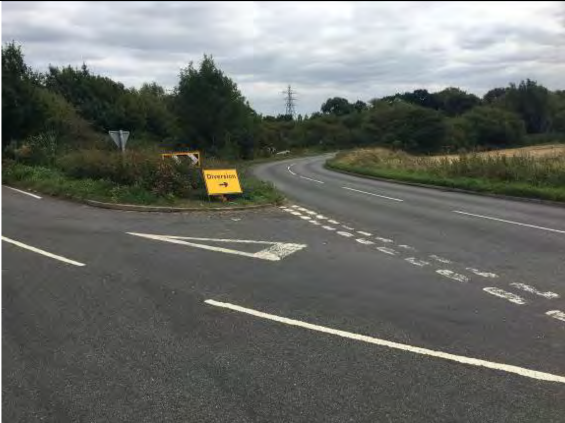
Image 2 – Existing yellow backed chevron signs facing eastbound motorists are partially obscured by overgrown vegetation
