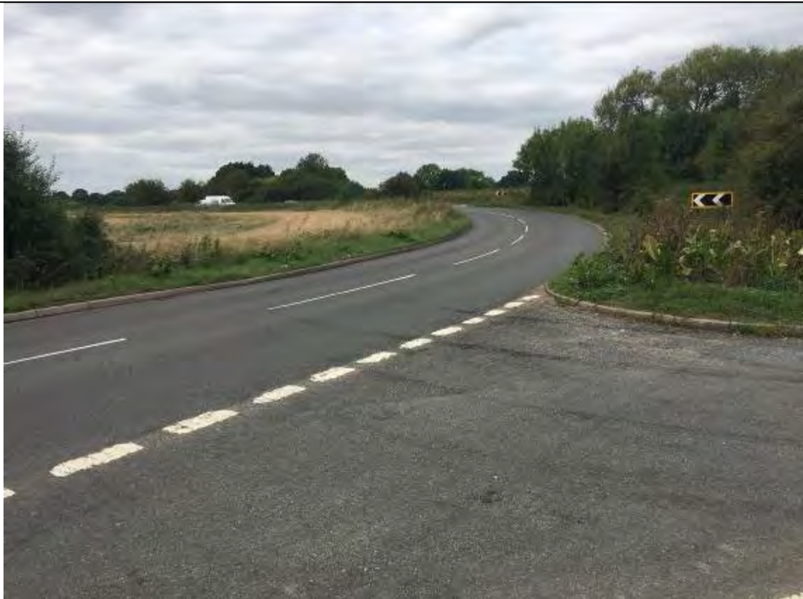
Image 4 – Existing yellow backed chevron signs facing northbound motorists are partially obscured by overgrown vegetation.
