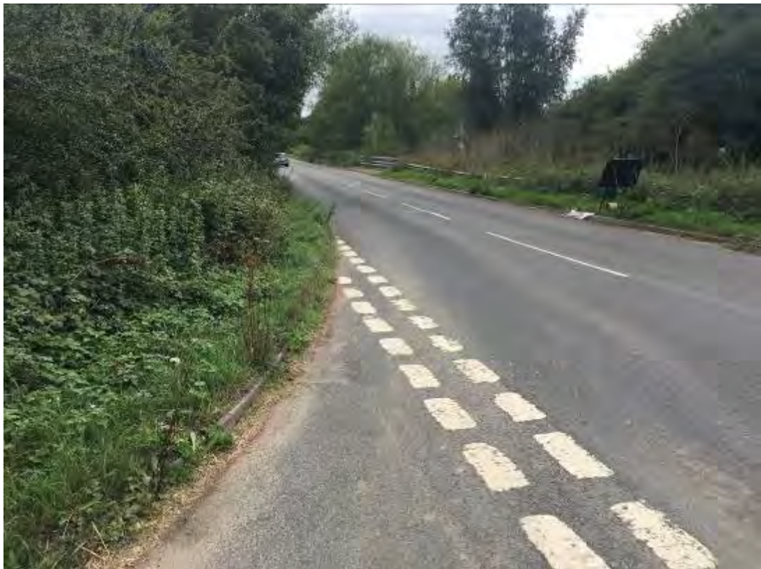
Image 7 – Visibility to the left from give way lines on Old Church Lane westbound approach (Southern Section) is partially obscured by overgrown vegetation.
