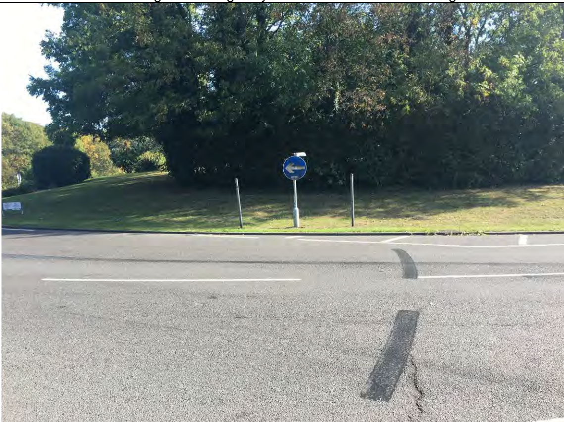
Image 3 – Chevron sign is missing from sign posts on the eastbound approach
