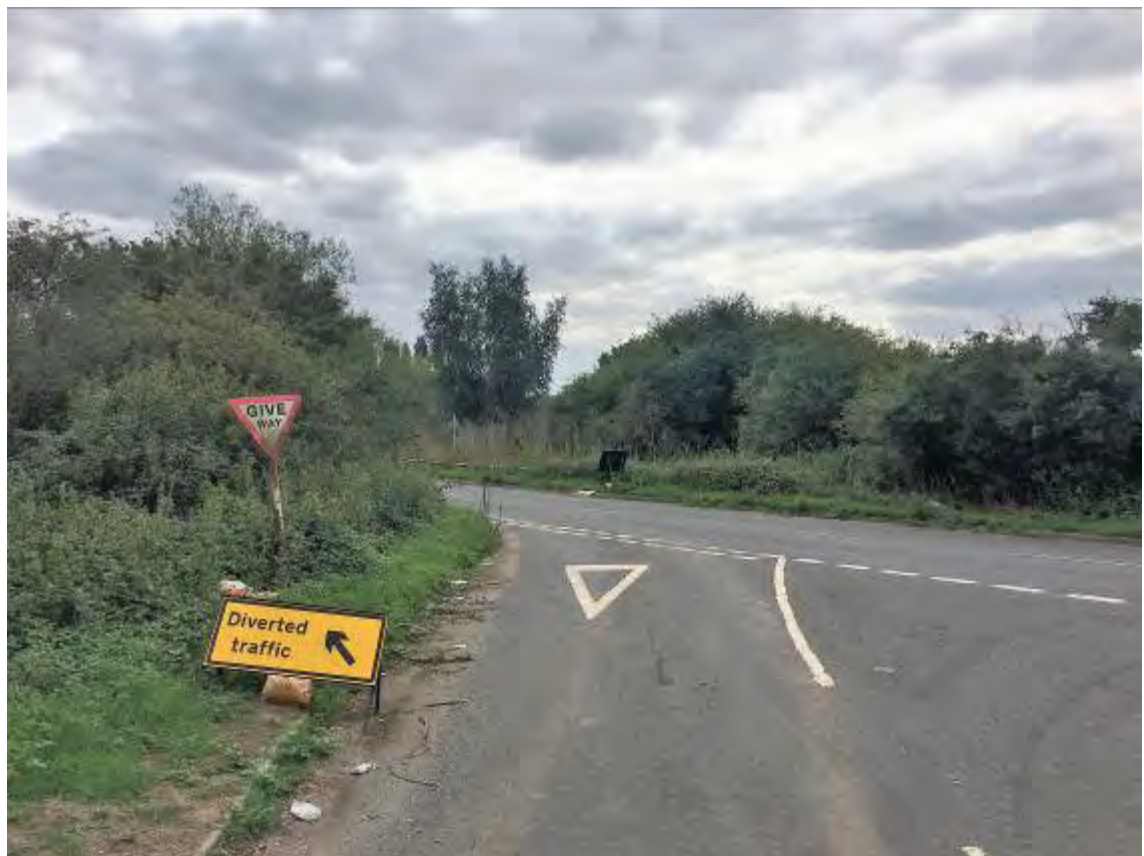
Image 5 – Existing 'Give way' sign on Old Church Lane westbound approach (Southern section) is partially soiled / dirty and the sign post appears to be rusty.
