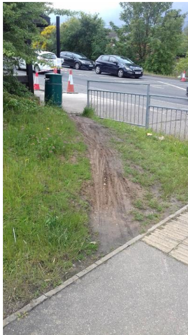
RSA1 Image 9 – Worn track adjacent to Bus Stop
