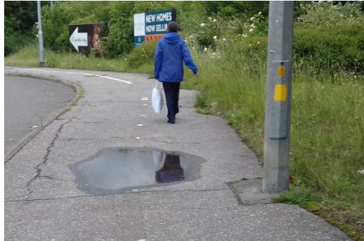
RSA1 Image 5 – Standing water within existing facility
