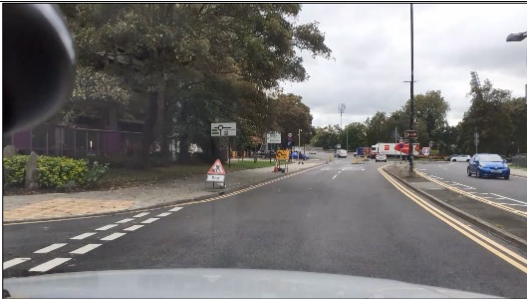
Image 4 – A1099 Victoria Road South, southbound approach Trees obscuring signs to nearside
