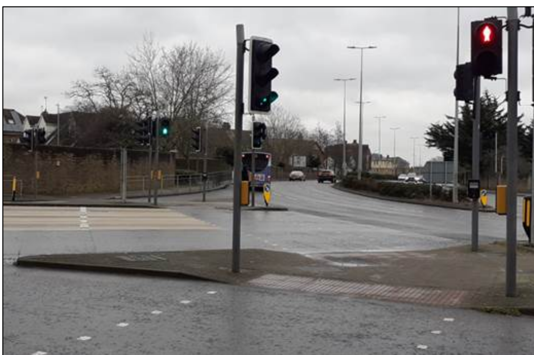
Image 5 – A1060 Rainsford Road (W) – looking south to north – Pedestrian signal head 'see-through'
