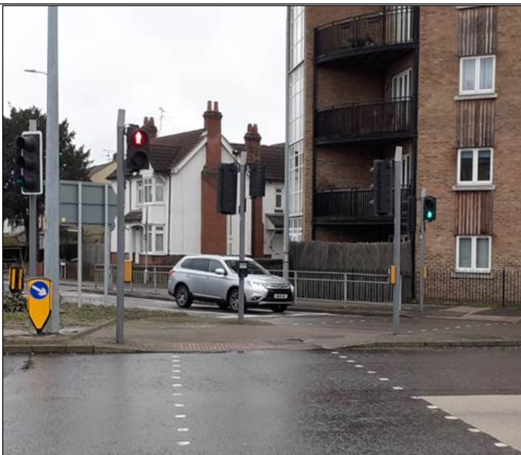
Image 6 – A1060 Rainsford Road (W) – looking north to south – Pedestrian signal head 'see-through'
