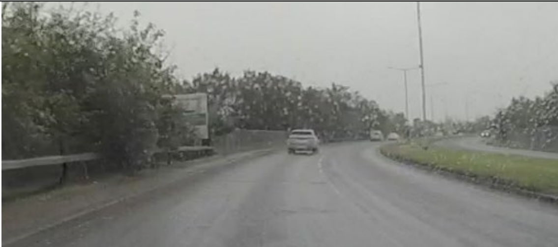
Image 1 – ADS sign obscured by vegetation. (southbound approach)
