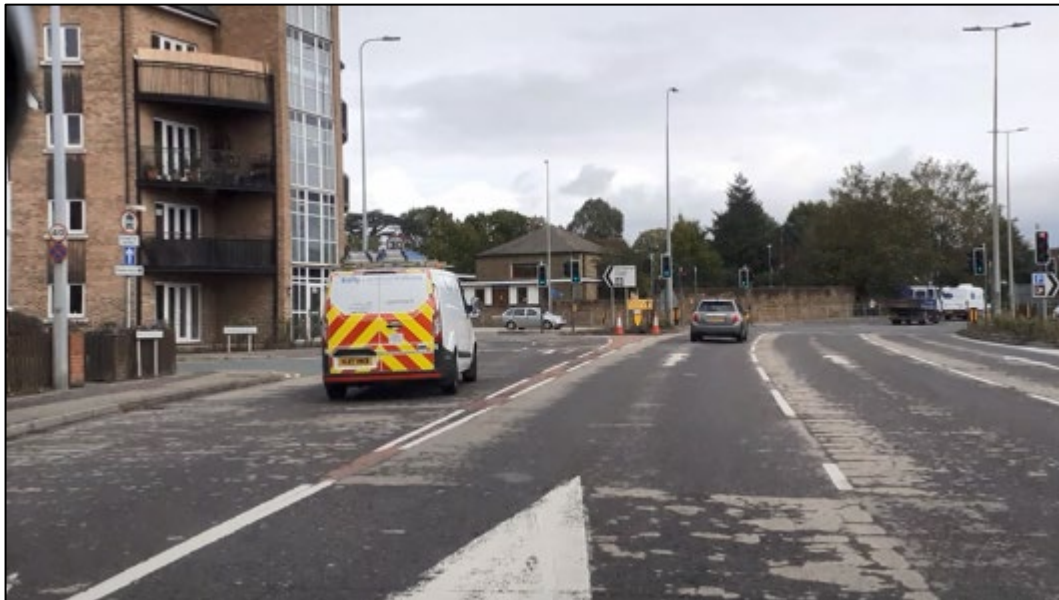
Image 1 – A1060 Parkway, northbound approach to junction. Note deterioration of high-friction surfacing and poor conspicuity of road markings.
