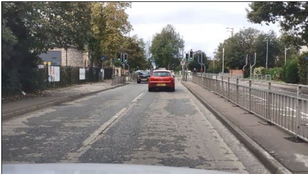
Image 7 – A1114 Princes Road westbound approach to Toucan crossing – poor condition of high-friction surface, poor conspicuity of road markings, and nearside trees compromising forward visibility
