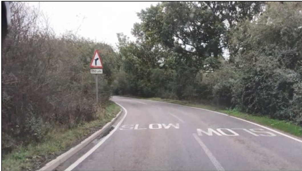
Image 3 – Boreham Road southbound worn centre lines and restricted forward visibility through left/right bends
