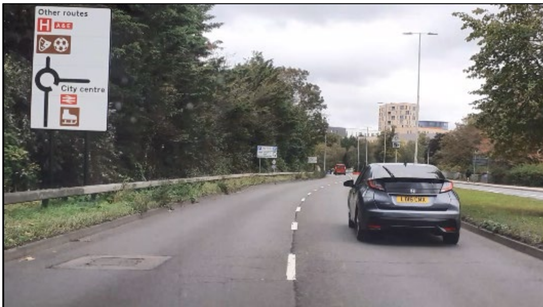
Image 1 – A1060 Parkway westbound approach. Note faded 'Roundabout Ahead' warning sign in central reservation.
