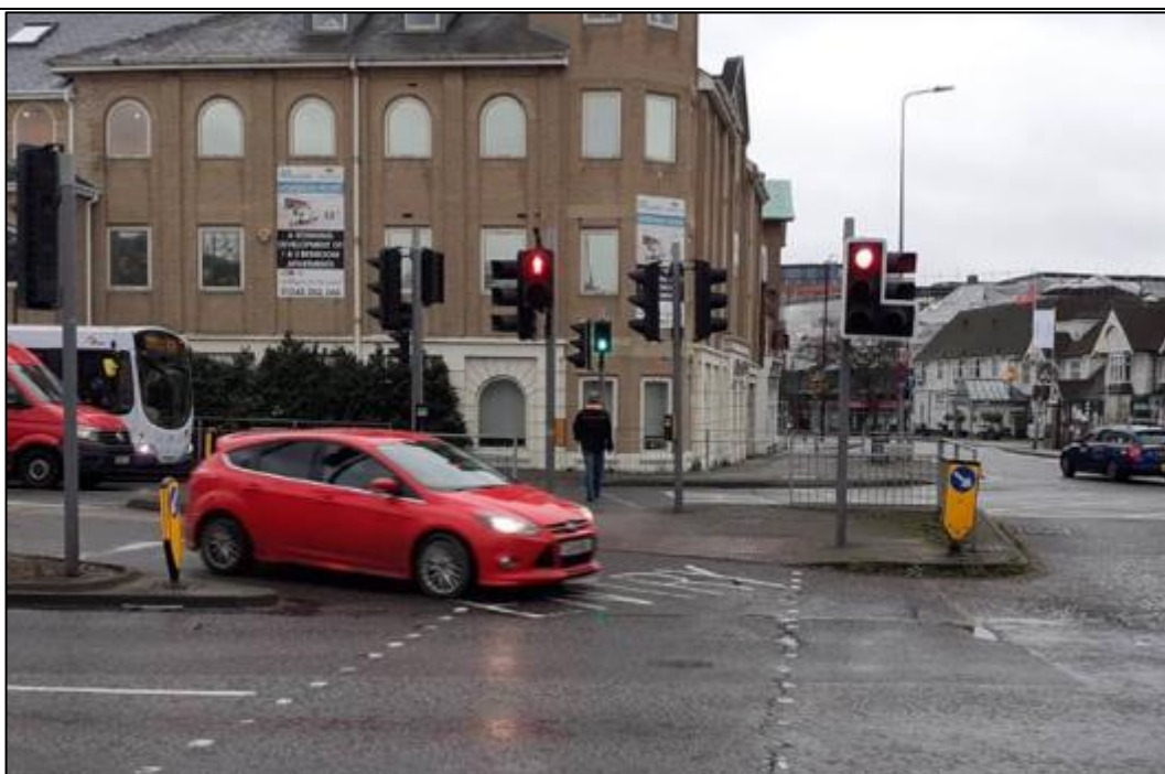
Image 4 – Pedestrian crossing, Parkway (N) - pedestrian signal head 'see-through'
