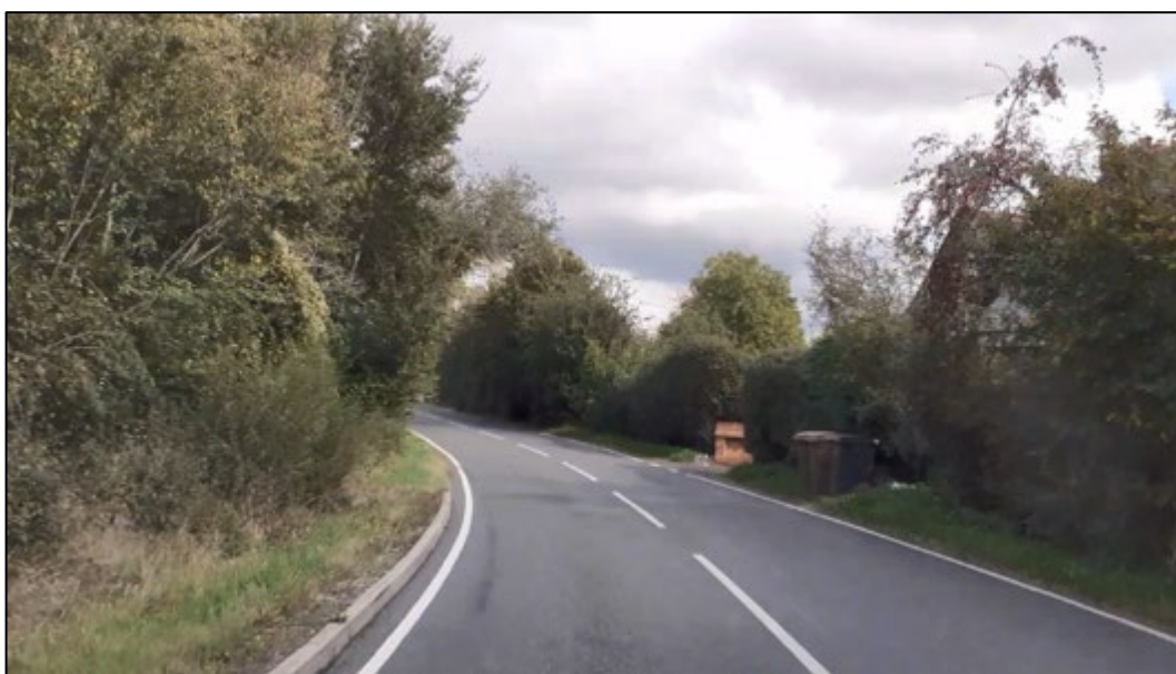
Image 6 – Cranham Road eastbound (opposing direction to Image 5 above) Note: locked tyre marks swerving to nearside and restricted forward visibility through bend
