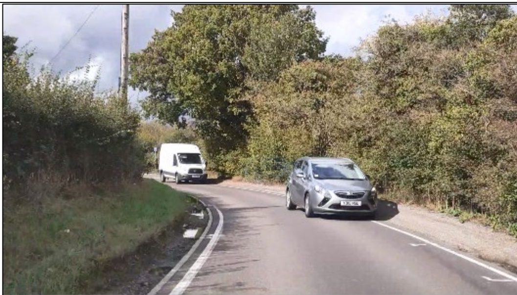
Image 7 – Boreham Road northbound verge erosion/incursion to both sides and limited forward visibility through narrow bend
