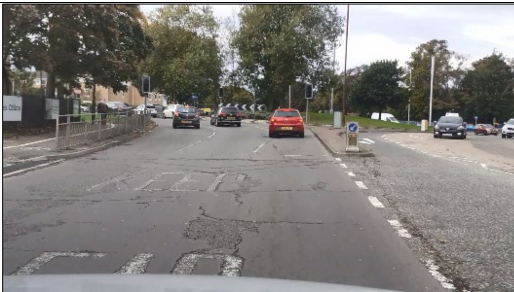
Image 2 – A1114 Princes Road, approach to Give Way lines at roundabout. Note poor conspicuity of road markings and overhanging trees to nearside.
