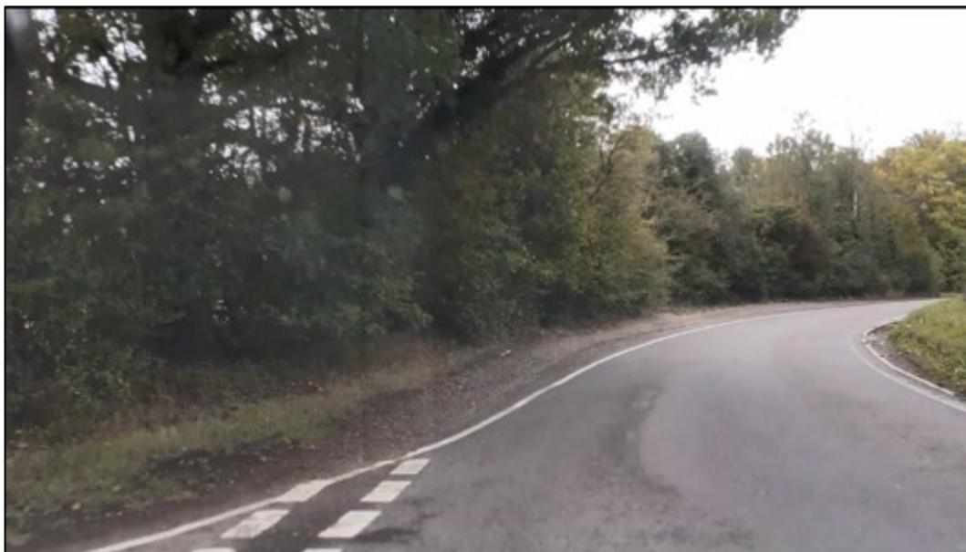
Image 4 – Boreham Road southbound, bend at j/w Birds Farm Lane (opposing view to Image 7) verge erosion/incursion to both sides and limited forward visibility through narrow bend
