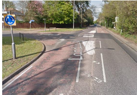
Figure 3 - Degraded condition of roundabout in 2019
